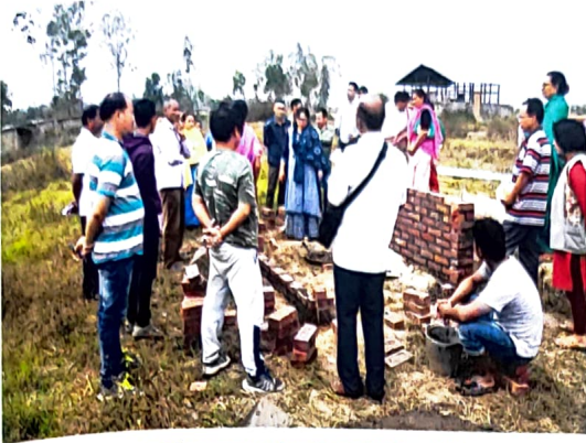
Demonstration on construction of Bokashi Piggery
