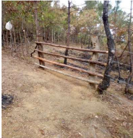
Fig 6: Entrance gate to mithun range constructed in the range
