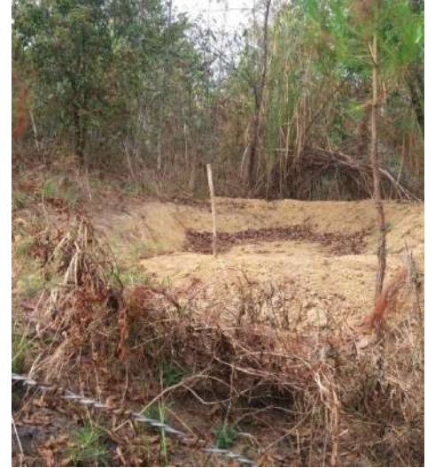
Fig 5: water reservoir constructed at
